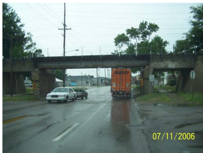
Green St. @ RR Bridge Near 4th (WB)
